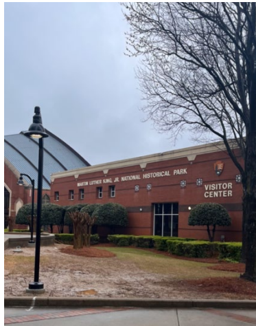
Fig. 5.20 Picture: Visitor Center
