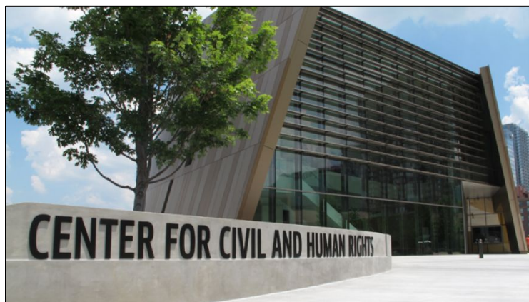
Fig. 5-26 Center for Civil and Human Rights Building
