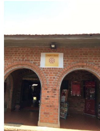
<Figure 49: The entrance of Dakshina chitra>
