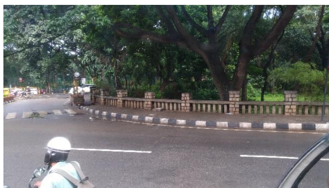
<Figure 9: Road with sidewalk>
