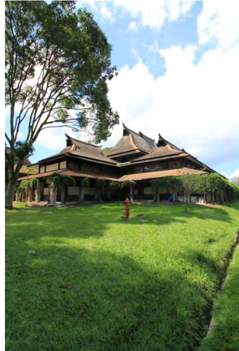
Fig.4 The old building of Civil Engineering department
