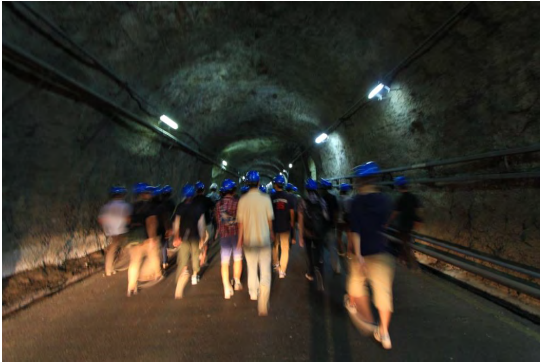
Fig.18 A long tunnel to enter the hydropower plant
